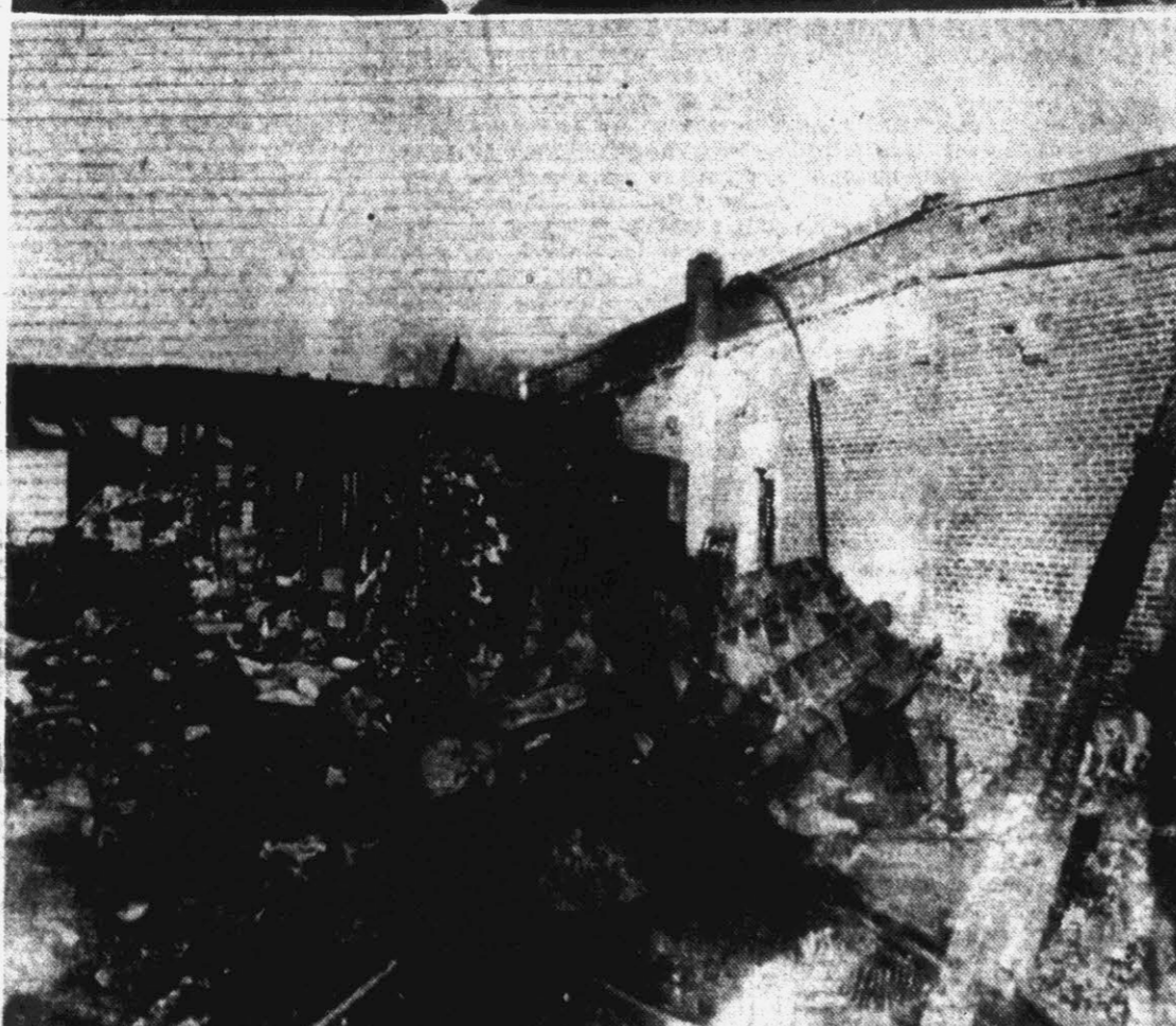
All that remains of the Carolina Sales Corporation which was gutted by a two alarm midnight fire Saturday is shown in the top photo. The bottom arrow indicates the area in which the fire was first seen by firemen when they arrived on the scene while the second arrow points to where the fire was first believed to have broken out before spreading to the side and becoming visible. Bottom picture shows an interior view of the smoking storage room and the fire wall which separated the sections of the building. Loss in the fire has been placed at $150,000 by company officials. Firemen fought a losing six-hour battle in an effort to save the structure, in snow and on frozen ground. (Reflector Staff Photo by Roy Hardee)
