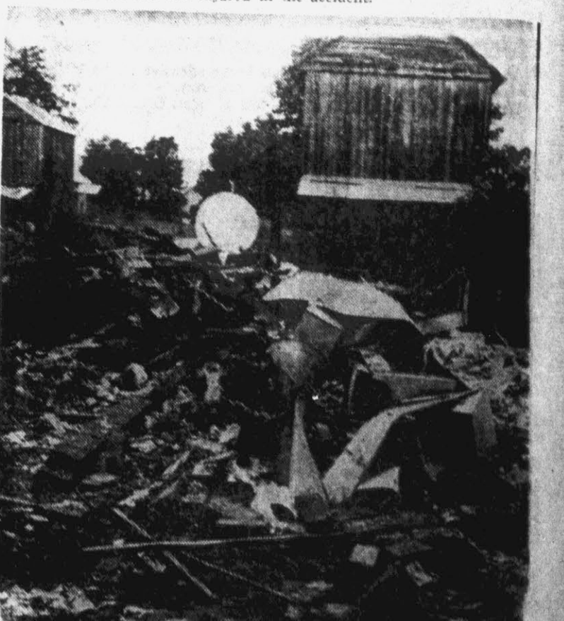
Part of the wreckage left in the path of a brief wind storm, that hit the L. M. McLawhorn farm near Winterville on July 27 is shown in the above picture. Tobacco barns filled with new tobacco were knocked down, out-buildings destroyed and heavy damage suffered by an area of about half a mile.
