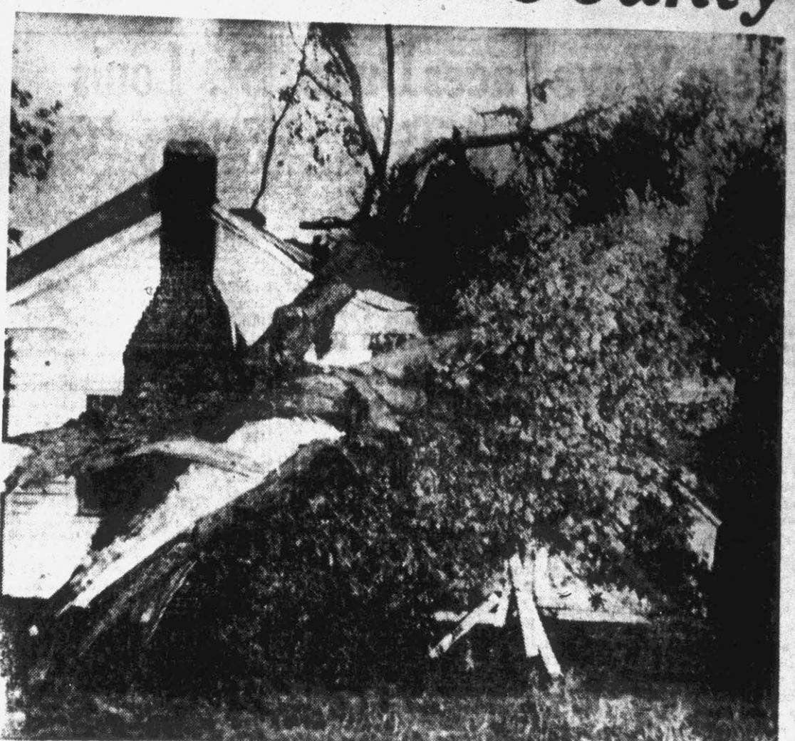
A destructive wind and hail storm struck a two-mile strip of farm land between Falkland and Fountain on May 12th. Property damage was heavy over the region with tobacco barns, power lines, torn down as well as trees uprooted and houses damaged all over the area.
