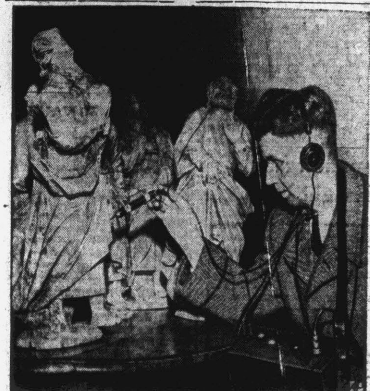
WORM-LISTENING DEVICE —An engineer at Leverkusen, Germany, tests a microphone and amplifier that magnifies sound 10,000 times, can locate tiny worms gnawing in wood.
