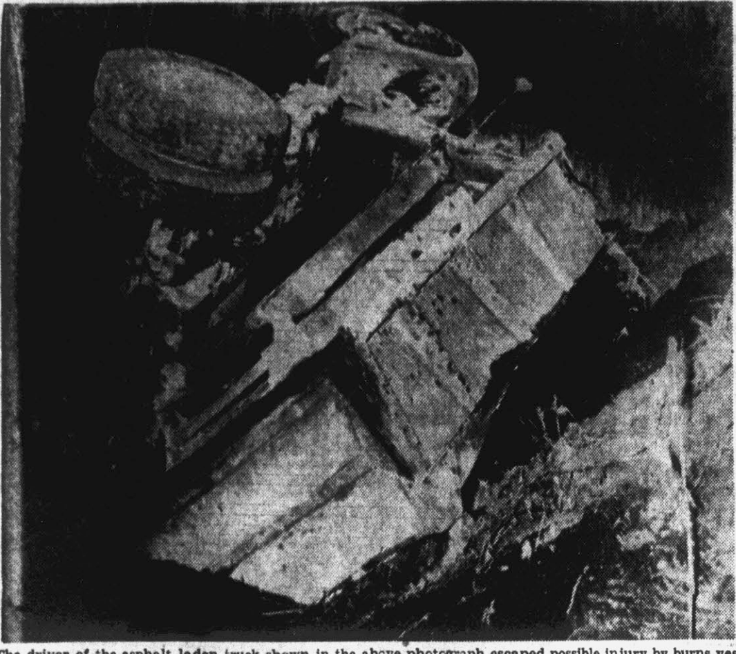
The driver of the asphalt laden truck shown in the above photograph escaped possible injury by burns yesterday afternoon when his truck left the Patoelus highway and turned over into a canal. The reason given for the accident was a blow-out of one of the tires. Patrolman Deiton E. Perry, who investigated, stated that the tire was "worn down to the fabric." (Photo by D. E. Perry, SHP).
