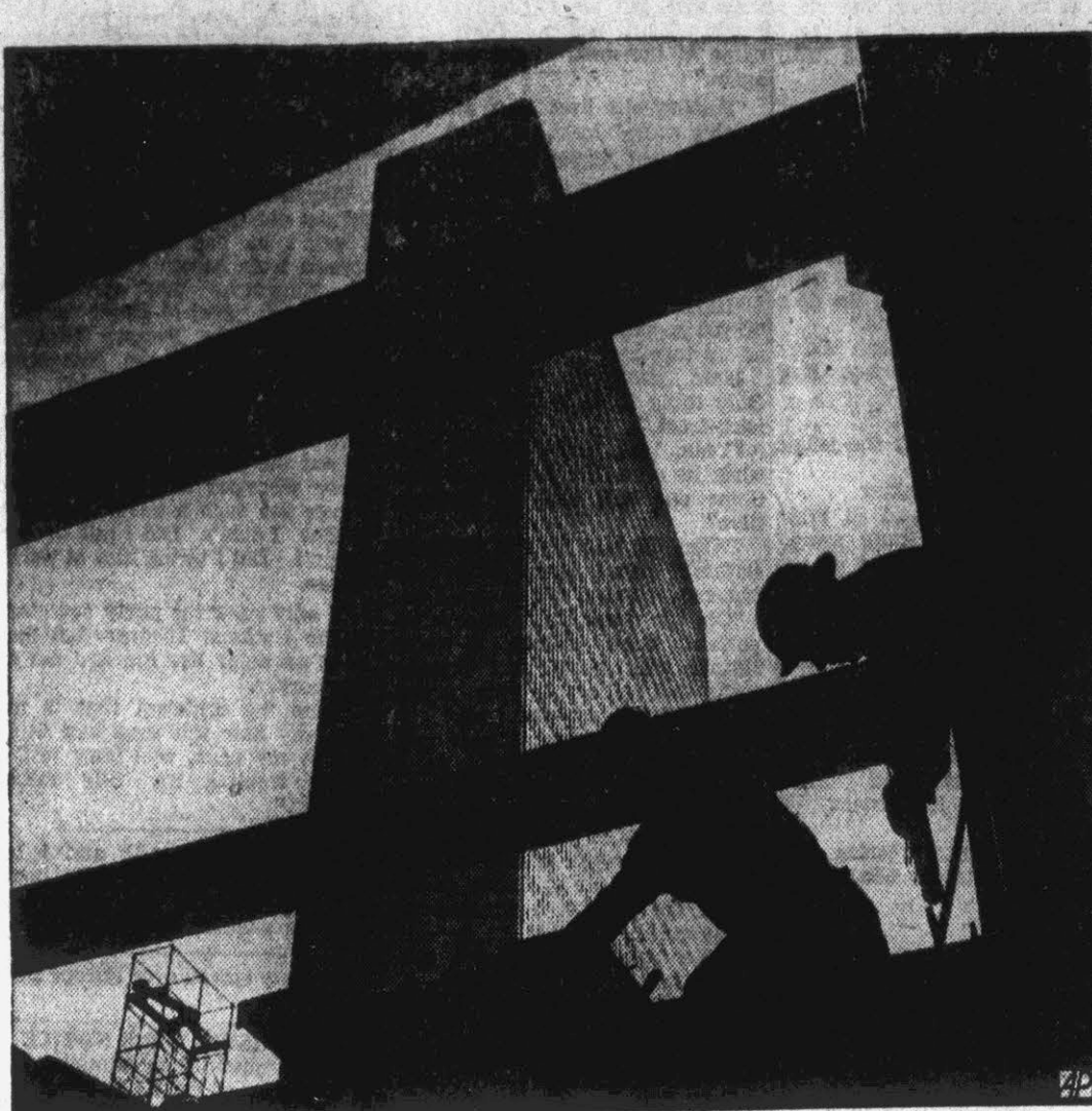
IN THE SHADOW OF THE U. N. — Silhouettes of two riveters frame United Nations building in New York working on steel framework of parking site for U. N. delegates, employes.
