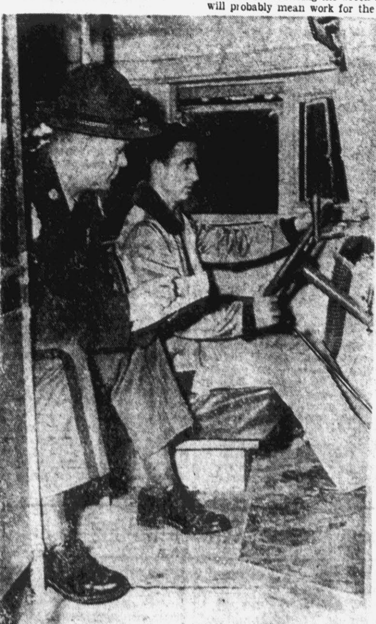
In addition to their regular highway patrols, the Pitt county patrolmen must inspect all of the Pitt county school bus fleet each month to determine if they are in top operating condition. In the above picture, Patrolman Ernest Guthrie of Farmville, observes Edward Duck of Winterville, a bus driver as he operates on one of the county's buses.
