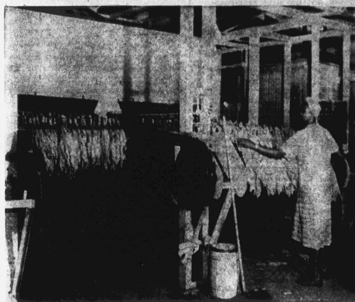
Here hands place the sticks of tobacco received from the hanging room on racks, and send them to the redrying room where they are kept for an hour. The process ranges in temperature from 175 to 210 degrees.
