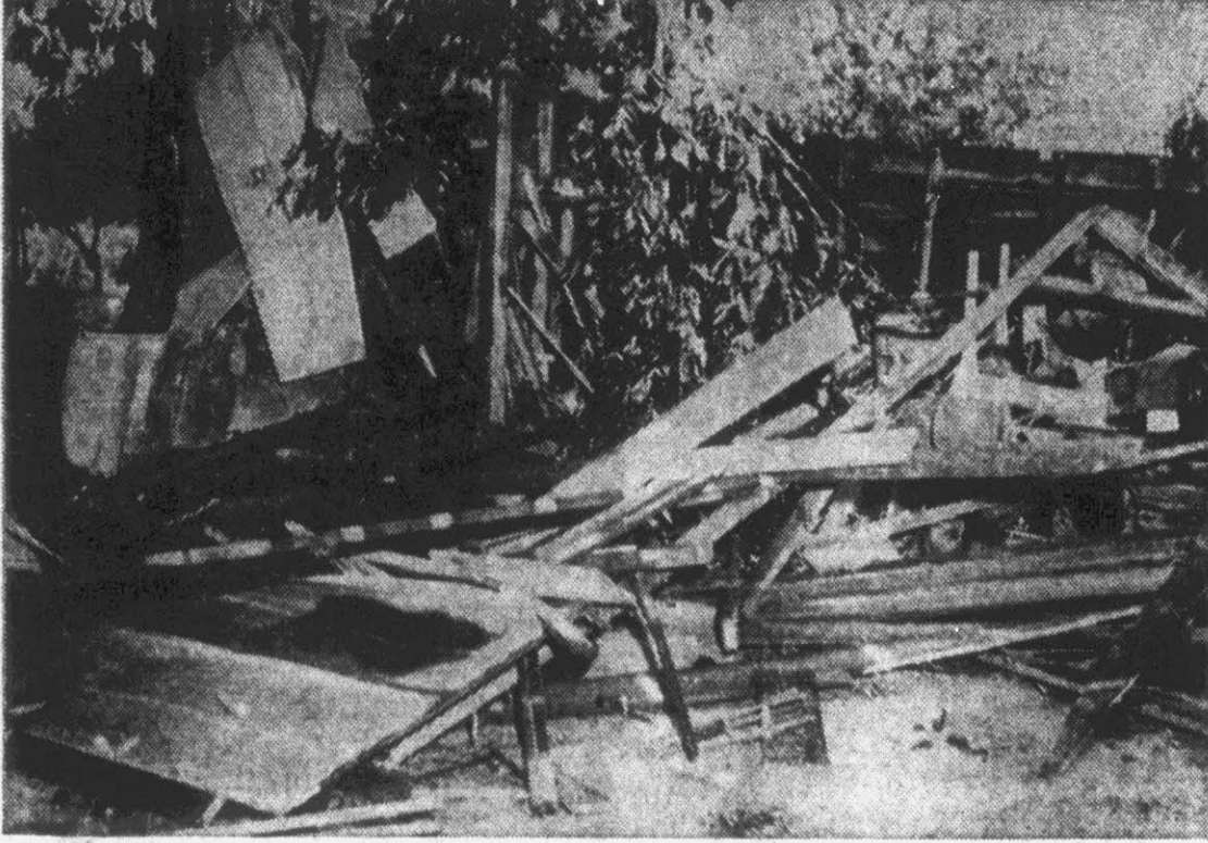
Splintered lumber and crumpled tin is all that is left of a wash house belonging to L. M. McLawhorn which was destroyed by the tornado yesterday afternoon. Wreckage and contents of the building was scattered over a wide area. Limbs were knocked from several trees, tin ripped from the roof of a nearby house, two large trees uprooted. Power lines in the area were put out of commission.
