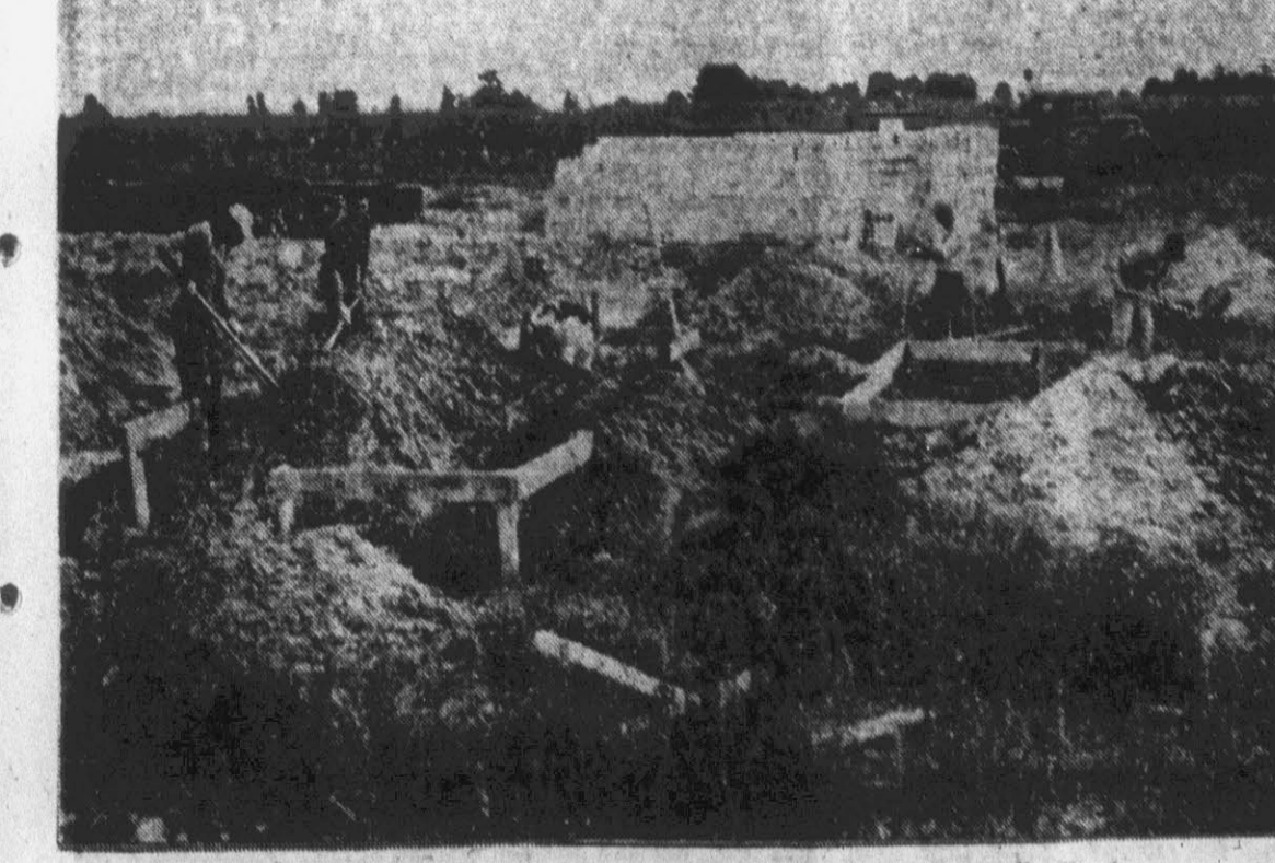
With the foundation laid, workmen are shown working on the Nurses home now being built behind the new hospital. A total of $85,000 is expected to be spent in constructing the building and an additional $40,000 for equipment. In the background a truck unloads some of the steel to be used in building the two-story structure. The majority of the materials for the building have been ordered and are expected to arrive at the site in the next few weeks. (Reflector staff photos by Roy Hardee.)
