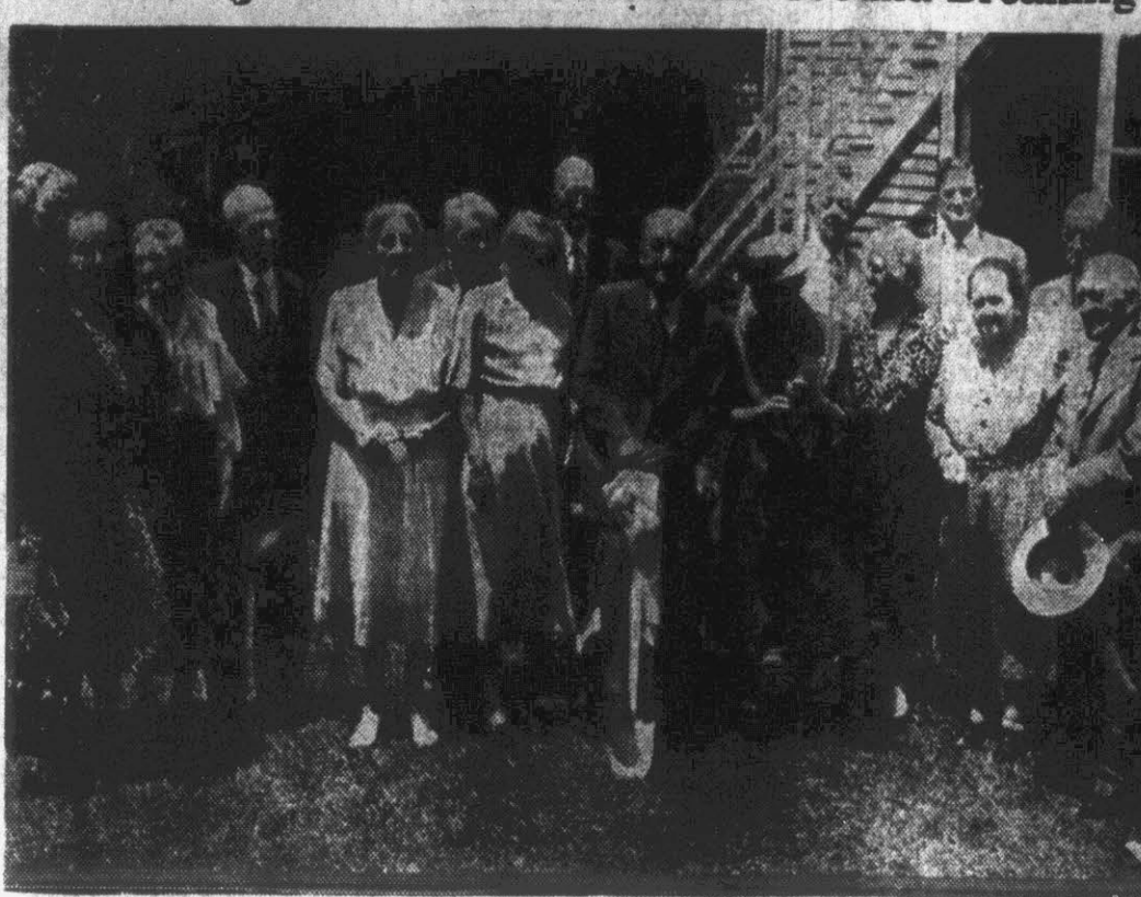
Mr. W. R. Smith, the oldest member of Jarvis Memorial Methodist church pauses just as he starts to dig the first shovel of dirt to start the construction of the new educational building at the church at ground breaking services held this morning. The new building will join the rear of the present educational building and extend to the James house. With Mr. Smith in the picture are the other members of the church who are eighty years and older. Each of the members took turns in the ground breaking. (Reflector staff photo by Roy Hardee.)
