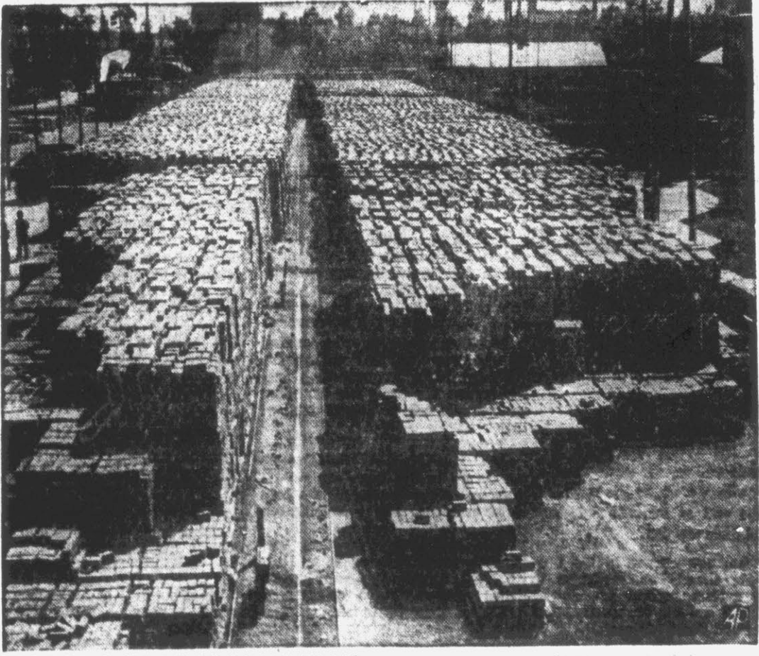
MODERN TRANSFORMATION—Bricks processed from rubble await shipment from a factory at Frankfurt-on-Main, Germany, for use in reconstruction of the war-damaged city.
