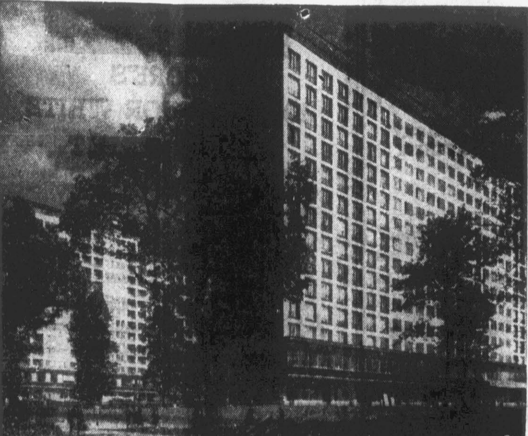
THE NEW GERMANY—Arising from the rubble of bomb-battered Hamburg, Germany, these modern 15-story apartment houses were built in 1949 to ease the city's housing shortage.
