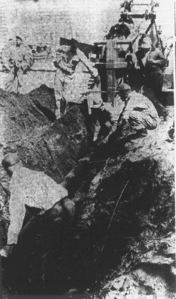
The first step in the laying of the tile lines for the draining of a field is the placing of the heavy metal outlet from which the water will flow. Here workers place the outlet in place. The tile is then laid in foot sections and covered with dirt. An average of over 2,500 feet of tile can be laid daily.
