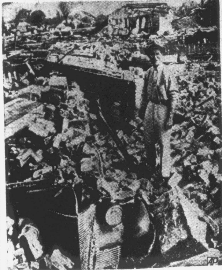
Here is some of the wreckage left by twin tornadoes that struck four suburbs of Mobile, Ala., injured 14 persons and did damage estimated at $250,000. A. O. Smith, an employee of the Stallworth Pine Products Company, looks at the debris of a company warehouse in the Whistler community. Smith's automobile (foreground) is buried under the ruins. (AP Wirephoto).
