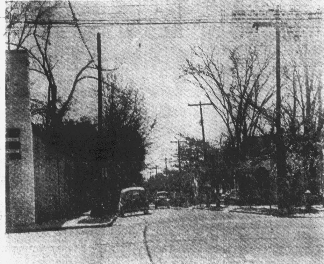
Not all of Greenville's traffic hazards are amply taken care of by traffic lights. In the top picture is shown a typical intersection in which four lanes of traffic travel. The vision of the drivers coming on the streets located next to the building is completely blocked until they enter the intersection. The building is located right on the sidewalk leaving only the sidewalk between the drivers and the intersection. Several serious wrecks have occurred at this intersection.
