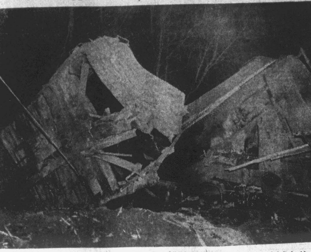
Freight cars as well as other debris were dragged from the right-of-way last night and left beside the embankment as crews worked to clear wreckage and lay new track at the scene of the Norfolk and Southern freight accident. The hook in the smashed freight car at the left is from one of the huge derricks which were used in the clearing operations. The track was cleared for passage about 3 o'clock this morning, but it will take several days to clear all the wreckage from the scene. (Reflector photo by Roy Hardee).
