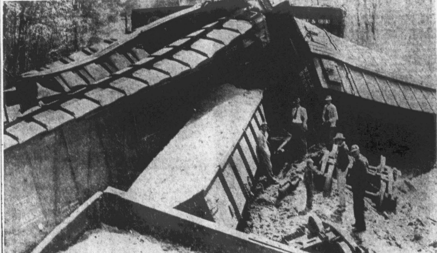
Twenty cars were derailed early this morning on the Norfolk and Southern railroad between Farmville and Bell Arthur in what was termed one of the worst wrecks the railroad has had. The photo above shows a portion of the wreckage along the road bed. Portions of the wrecked freight cars can be seen in the picture. (Reflector staff photo.)
