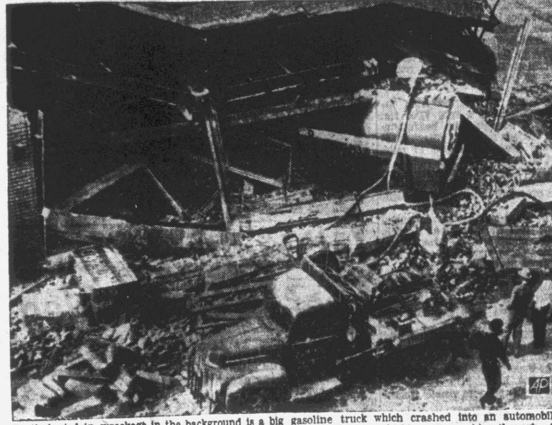
Partly buried in wreckage in the background is a big gasoline truck which crashed into an automobile show room at Lake Charles, La., and did $25,000 damage. The invading vehicle came smashing through after colliding with another truck. The roof of the building collapsed on the truck and several automobiles in the show room. Three persons received minor injuries. (AP Wirephoto).
