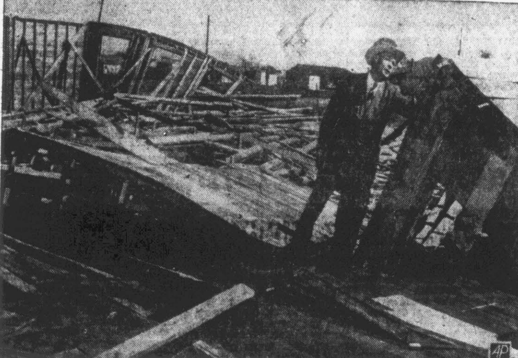
Pastor B. E. Smith stands amid the ruins of the First Baptist church at Elam, Tex., which was blown down by wind just as it was nearing completion. Members had worked at night to build the church with their own hands. When the storm struck, Pastor Smith was in the parsonage nearby reading the Bible—the sixth chapter of Joshua which tells of the walls of Jericho falling down. (AP Wirephoto).
