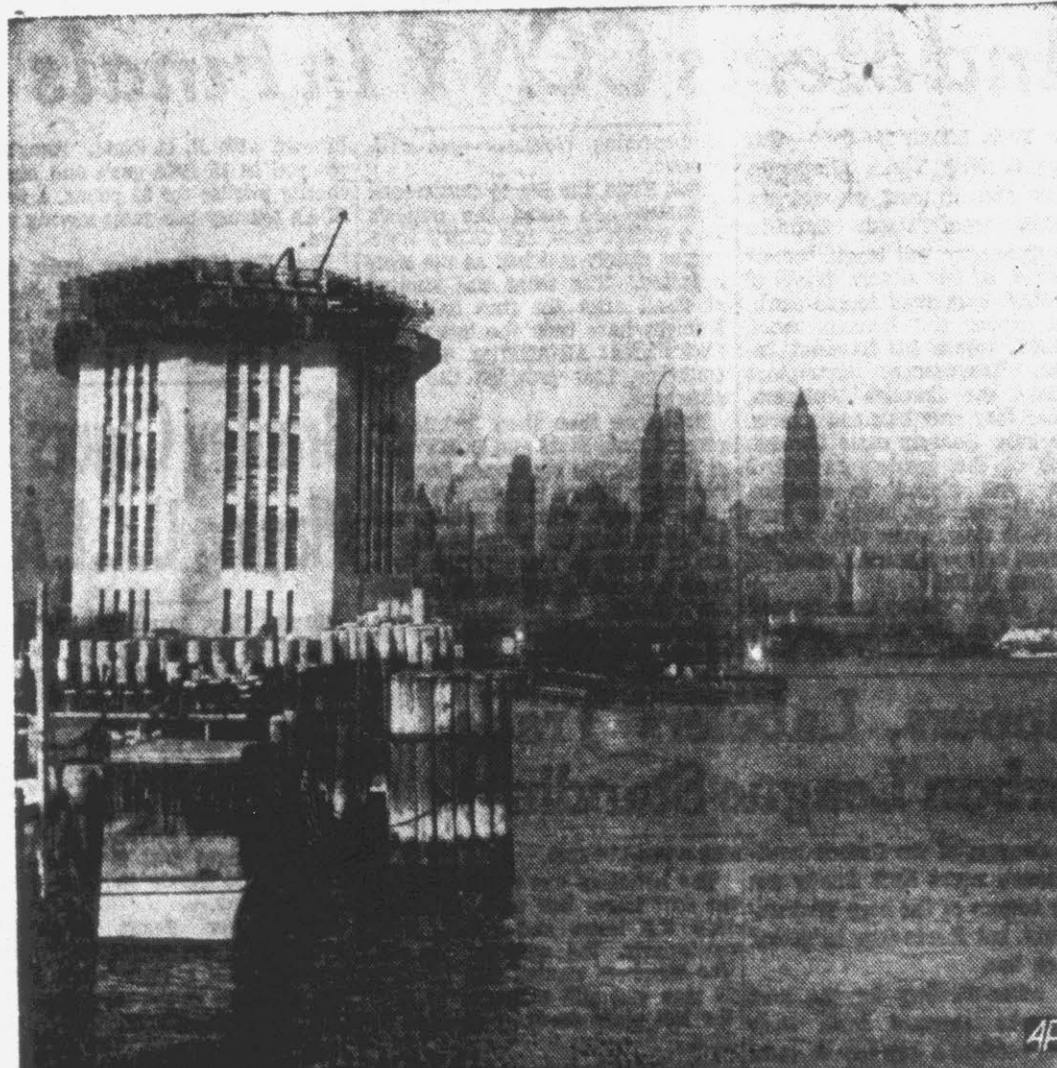
VENTILATOR FOR 9,117-FOOT TUNNEL —One of four ventilation buildings for New York's Brooklyn-Battery tunnel to open soon stands between Governors Island (foreground) and Manhattan skyline. $20,000,000, 9,117-foot tunnel links lower Manhattan with Brooklyn.
