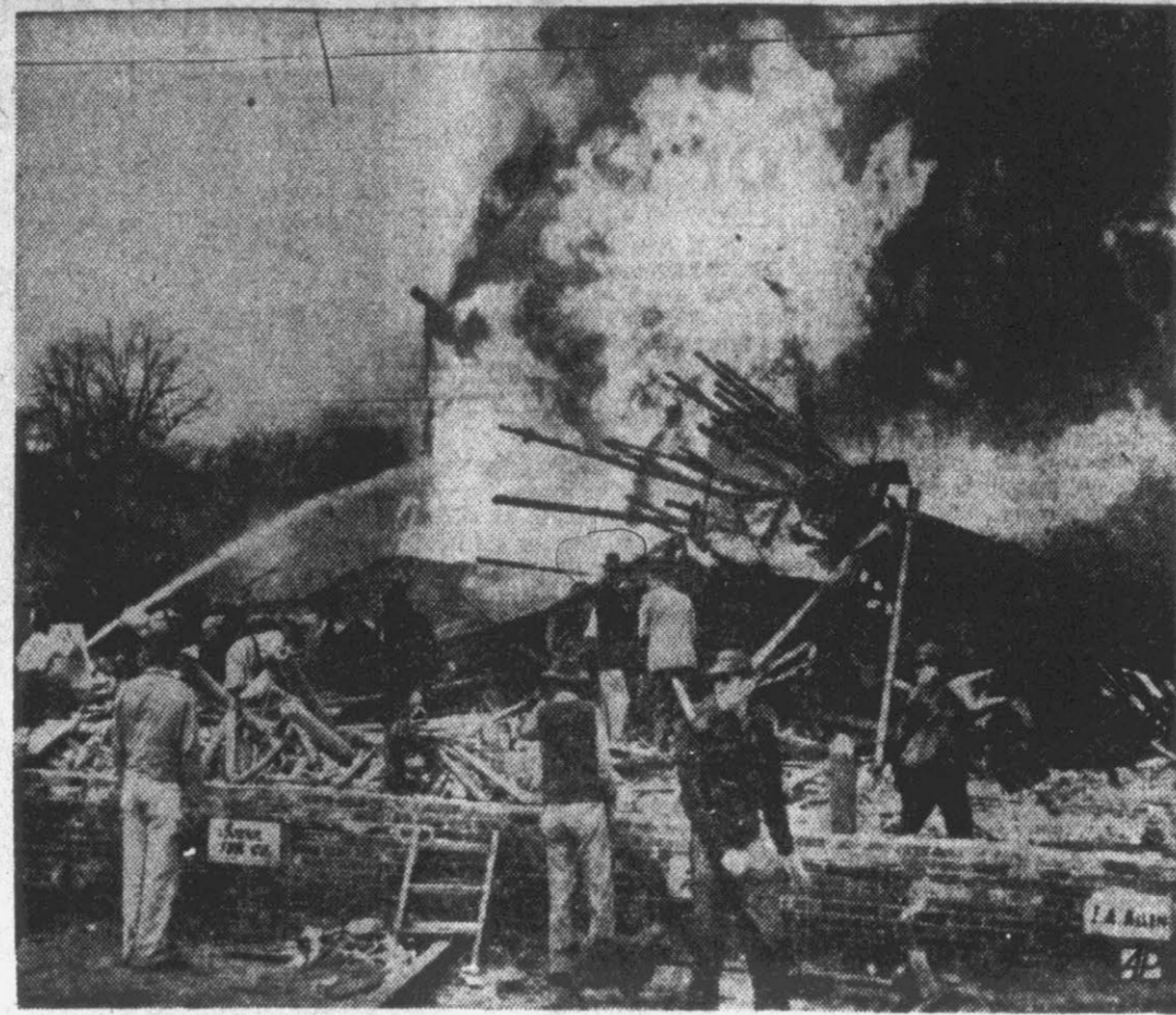
Flames sweep through part of block of business houses in Statesboro, Ga., March 18. Firemen and townspeople join to fight the blaze, which started after an explosion in a feed store. Three persons were injured. Damage was estimated at $300,000. (AP Wirephoto.)
