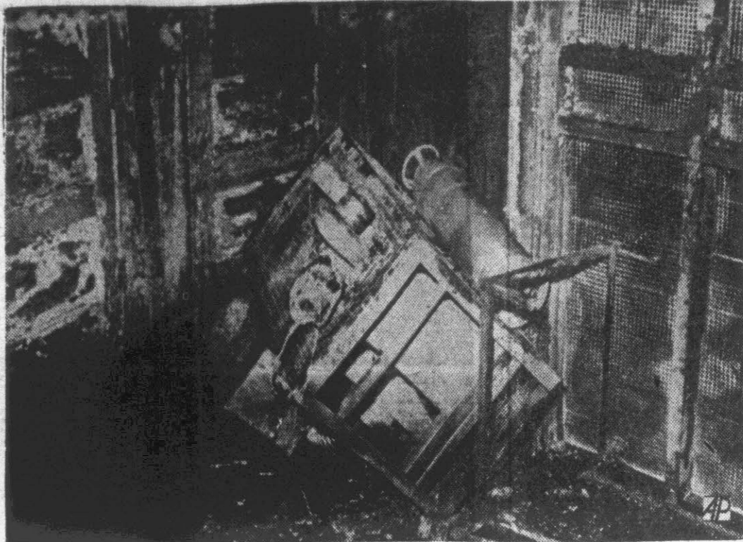
This overturned oil-burning stove is believed to have started the flash fire that swept through the Sandia Base guard house at Albuquerque, N. M., and took the lives of 14 military prisoners. Two other inmates were injured critically. At the right is the heavy wire mesh door leading to the inner cellblocks in which the prisoners were trapped by the flames. The charred doors at left open into solitary confinement cells which were empty when the fire broke out. The Sandia Base is a semi-secret assembly point for the atomic bomb. (AP Wirephoto).
