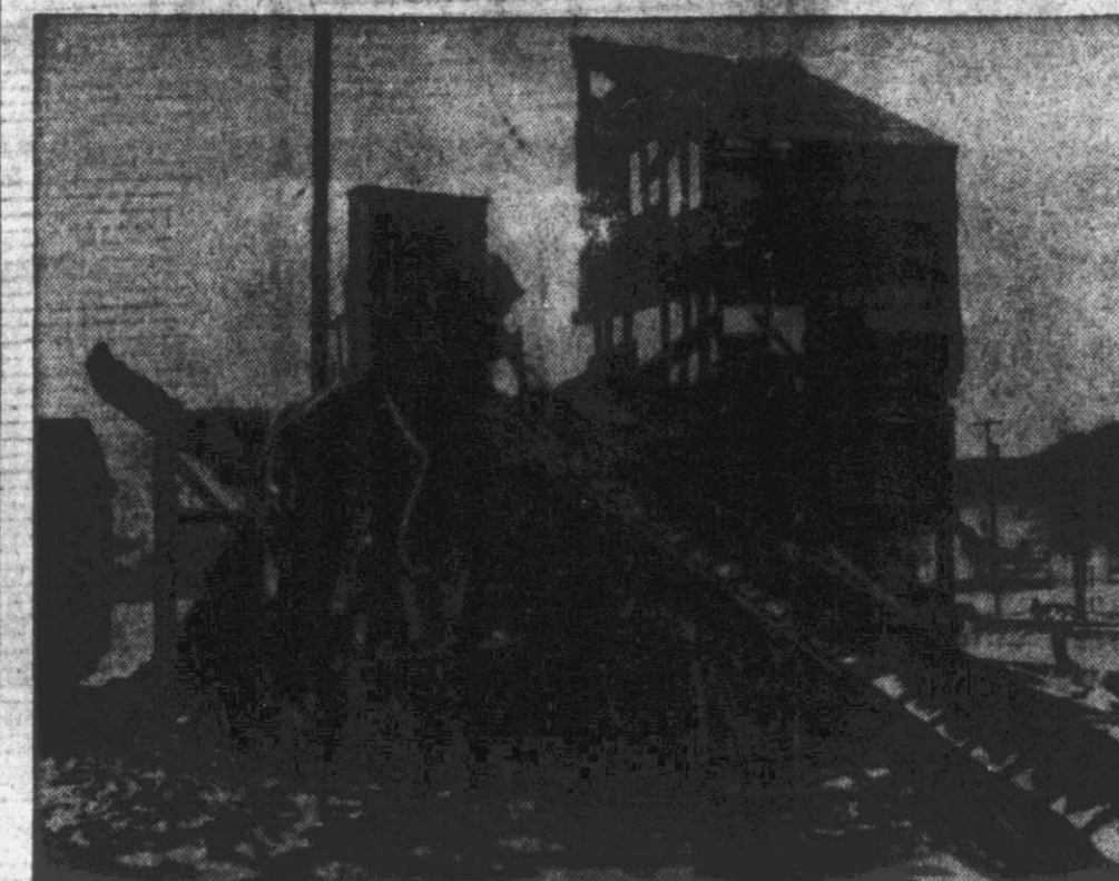
Police say this coal loading tippie used by non-union miners at Brookway, Pa., was wrecked by a dynamite blast set off by pickets. No one was hurt but the explosion shattered windows in nearby homes. Squads of union miners are roaming through the coal fields in attempts to close non-union coal mines. (AP Wire-photo).
