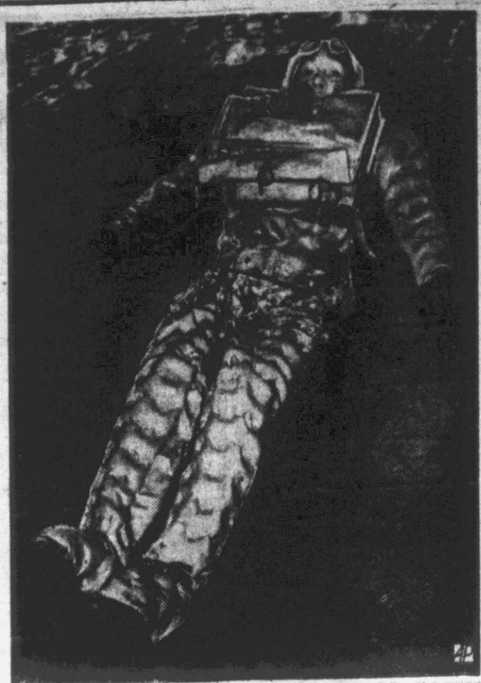
SUBMARINE ESCAPE SUIT —A new inflated submarine escape suit worn by a British Navy man at Portsmouth, England, holds a bulb which lights when immersed in salt water.
