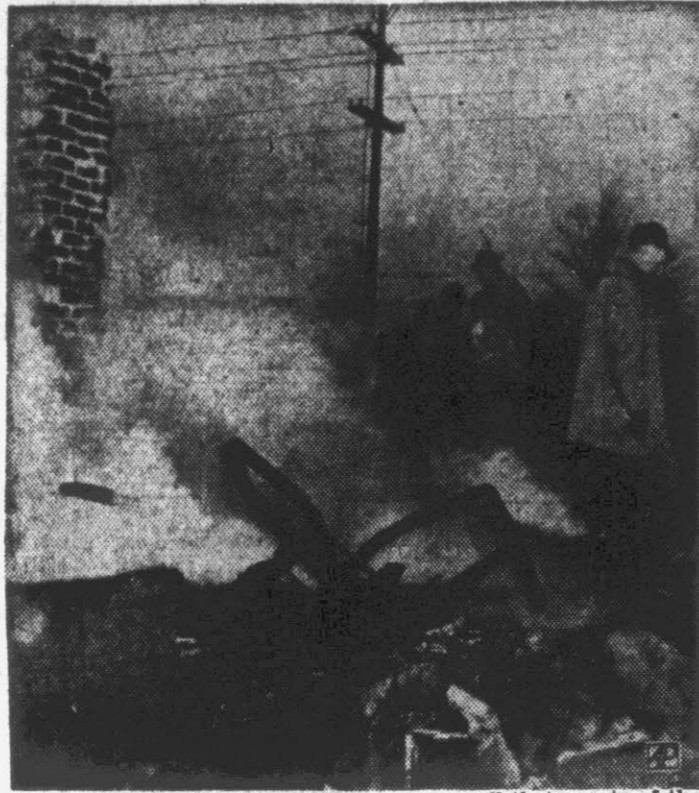
Charred and twisted bedstead and chimney are all that remain of the Emmett, Mich., farm home of Mr. and Mrs. Clarence Bethway where five of their 11 children were burned to death. The blaze started from an overheated coal stove trapping the five victims upstairs. The parents, grandmother and five other children escaped through windows. (AP Wirephoto).
