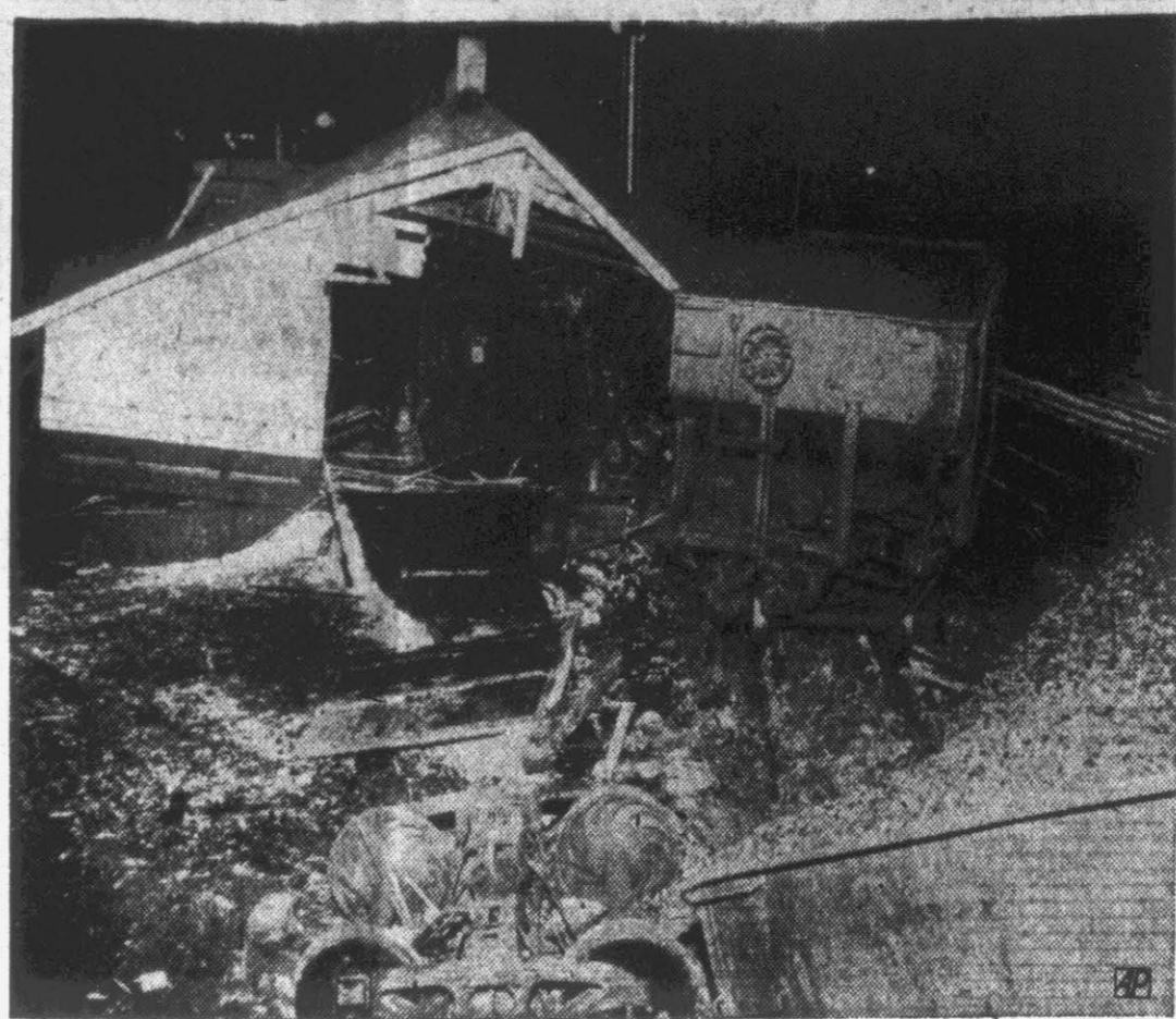
A gondola of coal hurtled from the tracks in the derailment of 17 cars of a Northern Pacific freight train and smashed into the railway station at North Branch, Minn. No one was injured, but the station was completely demolished. (AP Wirephoto).
