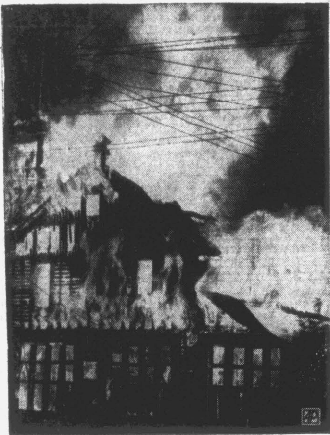
This raging fire is destroying the fire station at Albion, Pa. It was believed the flames started from an overheated stove. The building and all of the town's fire-fighting equipment were lost. Two nearby buildings caught fire and were damaged. (AP Wirephoto).
