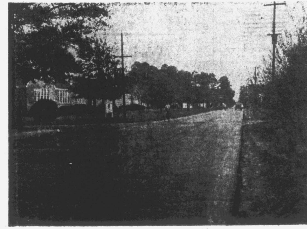
Pictured above is one of the broad new streets which the people of Winterville have had put down in their town during the past two weeks. All the paving was done by the footage payment of the property owners rather than through the levying of taxes or the issuance of bonds. The new paved streets of the town range in width from 18 feet to 40 feet.
