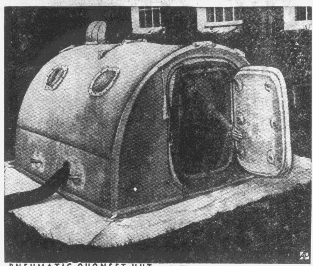
PNEUMATIC QUONSET HUT —This pneumatic quonset hut of cotton fabric, made for airmen stranded in Arctic, was developed by Air Materiel Command and U. S. Rubber Co. It has no internal braces and can be supported by 1½ pounds of air pressure, supplied by hand pumps. Designed to withstand 100-mile-an-hour gales, it is snowproof, waterproof, draftproof.
