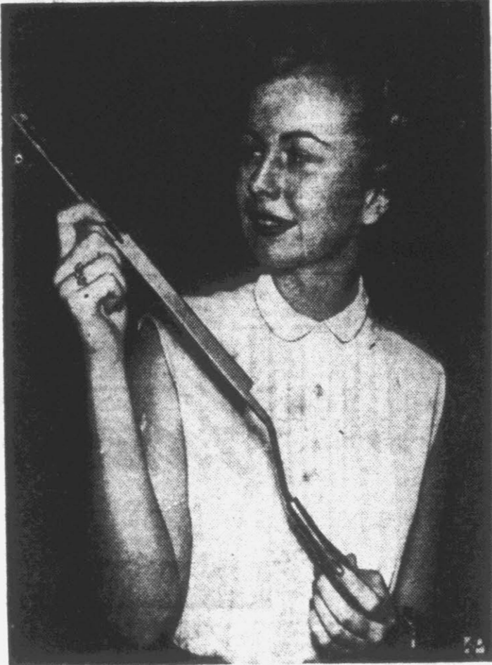
NEW USE FOR OLD BLADES—Ann Allhusen demonstrates at a New York hardware show how old razor blades may be fitted into a "grasshaver" for trimming grass and weeds.
