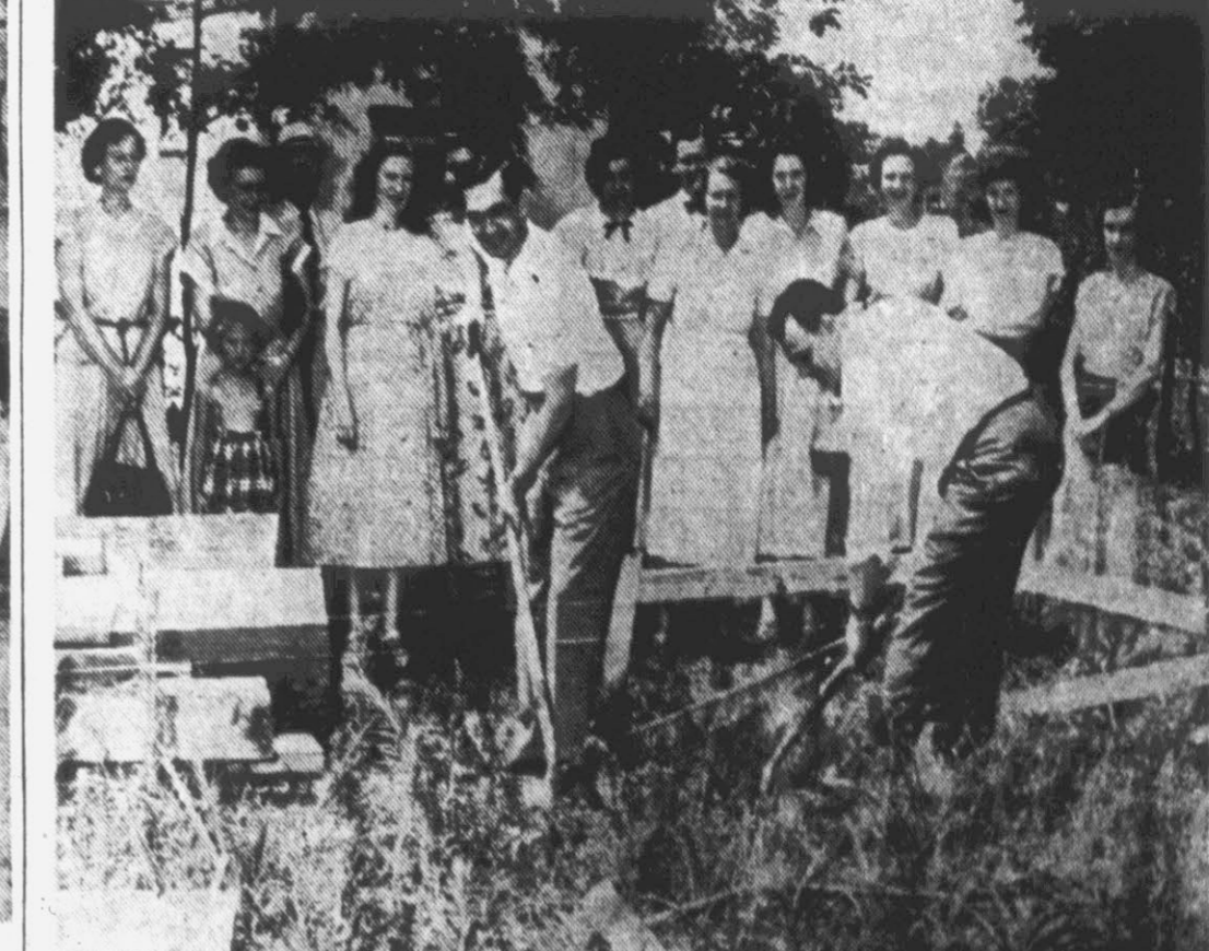
Earl Addler (left) commander of the Greenville V. F. W. post, and Ty Wagner (right) commander of Pitt County Post 39 of the American Legion lifted the first shovel full of dirt at the ground-breaking ceremony when construction on the O'Neal home was begun in June. Others who were active in forming the O'Neal foundation watch the ground-breaking.
