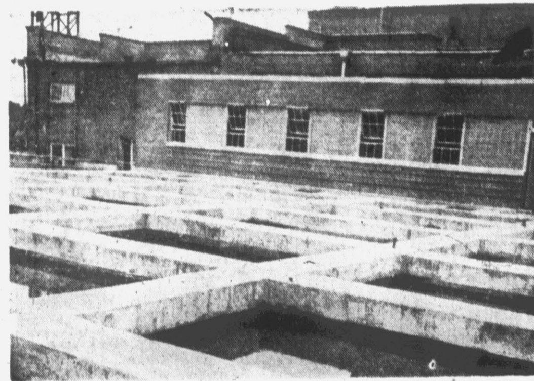
The filtering plant is one of the most important units in the process of treating the raw river water and turning it into clear pure water. Through this unit will pass a capacity of 3 million gallons of water in a 24-hour period.
