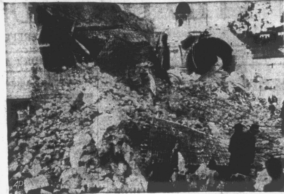
Ruins of the town cathedral at Ambato, Ecuador, are piled high in the street by the earthquake that killed thousands of people in 50 communities. Two hundred were reported killed in the fallen cathedral. The mighty quake destroyed many homes and left about 100,000 people homeless. (AP Wirephoto).
