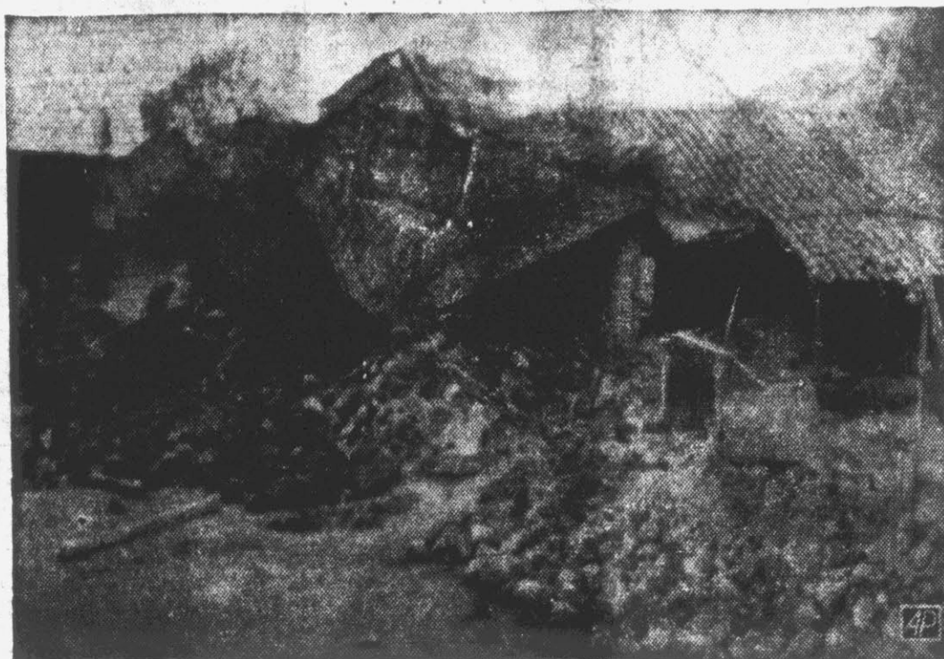
Here is a scene of devastation in the town of Pelileo, Ecuador, one of 50 communities destroyed by the earthquake that killed thousands last Friday. Survivors are digging into the ruins in search of dead and injured. Some estimates placed the number of dead at between 2,000 and 4,000. Many perished in Pelileo. (AP Wirephoto).
