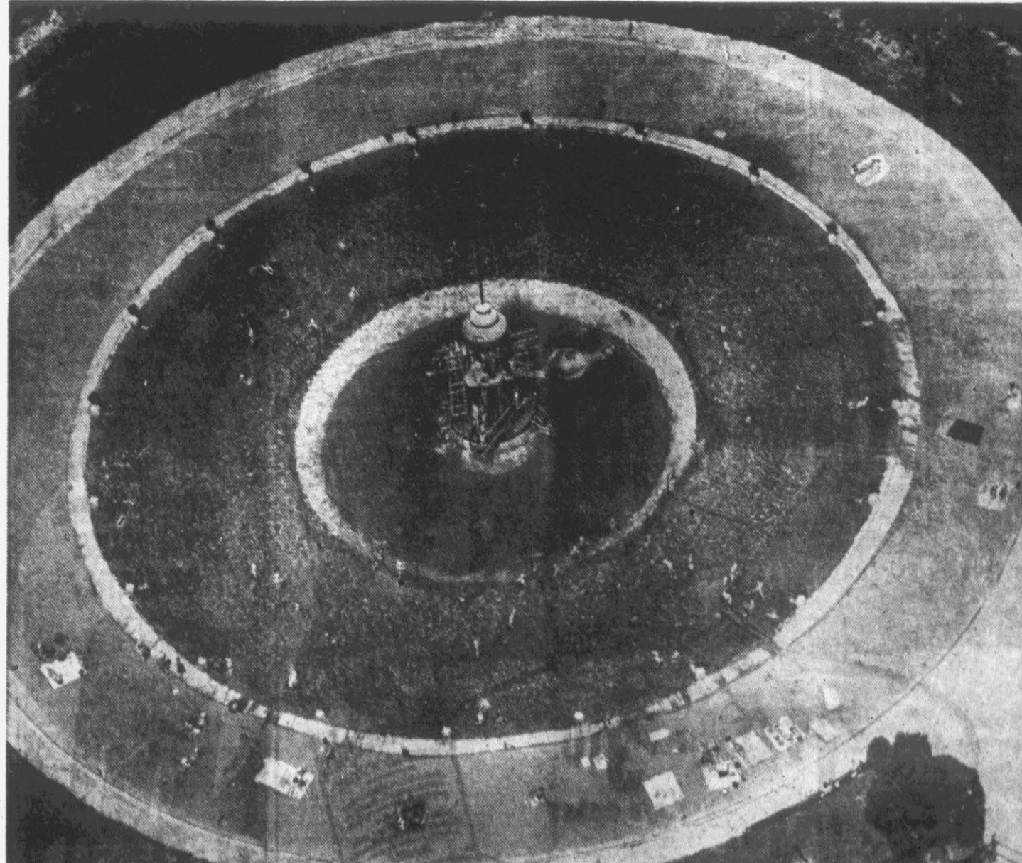
SERVES 1,798 IN TOWN OF 7,000 —Seashore Pool, in Lebanon, Ind., (population 7,000) can accommodate 1,798 persons daily. Center is 10 feet deep, with shallow water next, sloping up from 4 1/2 feet to a sand beach and greensward.
