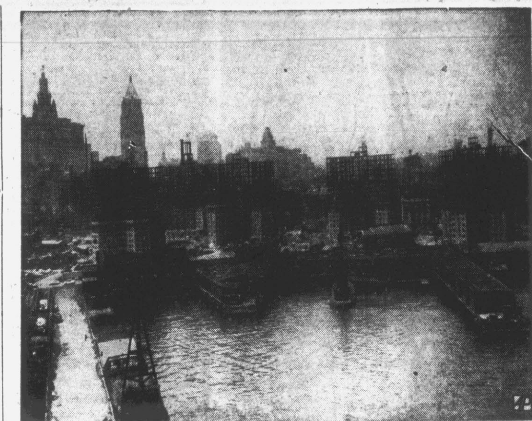
WHERE 1940 FAMILIES WILL LIVE —Steel skeletons of some of the 13 buildings in the Alfred E. Smith housing project rise on New York's lower east side. The buildings, of 16 and 17 stories, will cost $28,000,000, and, at low cost, will house 1940 families.
