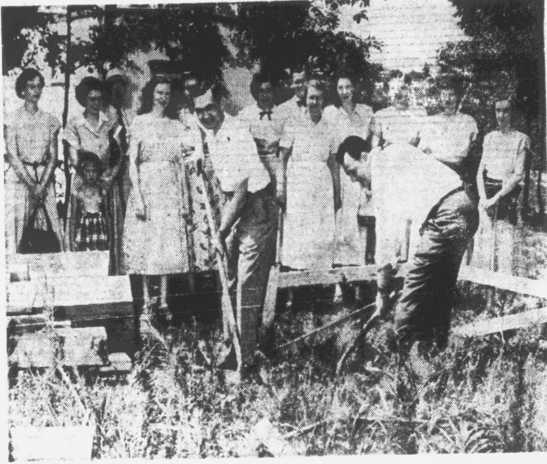
H. Earl Adler (left) commander of the Greenville V. F. W. post, and T. I. Wagner (right) commander of the Pitt county American Legion post are shown breaking the ground for the house to be built by the O'Neal Foundation for the mother and the widow of William Benjamin O'Neal who was slain last February. Watching the ground-breaking ceremonies are (left to right) Mrs. Godfrey Oakley, chairman of the Watson memorial fund of the Junior Woman's club, Mrs. Johnston Dees, secretary of the O'Neal Foundation, Mrs. White Shrine, J. S. Moye, treasurer of the O'Neal Foundation, Mrs. Dixon, mother of Mrs. W. B. O'Neal, Jr., Mrs. Kenneth Brown, president of the V. F. W. Auxiliary, Mrs. Larry Ave., member of the board of directors of the O'Neal Foundation, Mrs. C. B. West, Jr., and Mrs. Jesse Laughinghouse, chairman of the White Shrine O'Neal Foundation committee.
