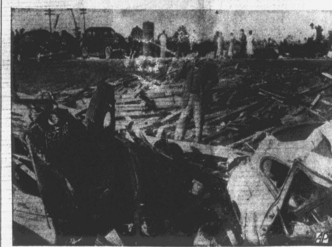
Two wrecked automobiles rest amid rubble after they were hurled 200 feet across highway (background) during the deadly tornado at Cape Girardeau, Mo. The car at left was owned by F. D. Shoulters (center) who was working in a restaurant that was demolished. He escaped with head injuries. The tornado killed 21 people, injured 112 and did damage exceeding $3,000,000 at Cape Girardeau. (AP Wirephoto.)
