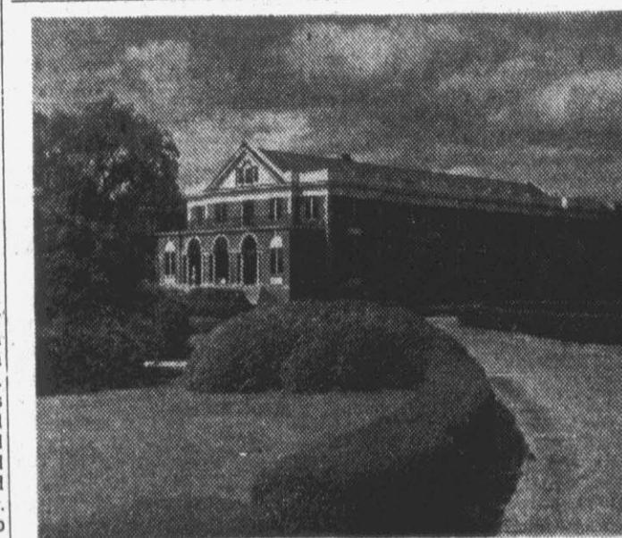
A program of building and improvements in present facilities will bring about many changes on the East Carolina Teachers College campus. The library (shown above) will be converted into a music building after the completion of a new library, which according to present plans will be located just west of the infirmary.
