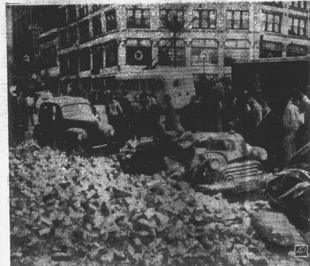
Fallen bricks from a shattered building crushed these automobiles on a street in Seattle, Wash., during the terrifying earthquake that jolted the Pacific northwest Wednesday. At least five persons were killed in the area, many were injured and property damage ran into the millions. (AP Wirephoto).
