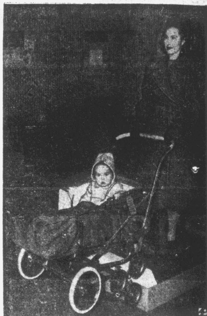
NO-BUMP PRAM —Small wheels attached to the rear axle keep baby's ride smooth even on stairs and street curbs in this carriage shown at the London Inventor's Club exhibition.
