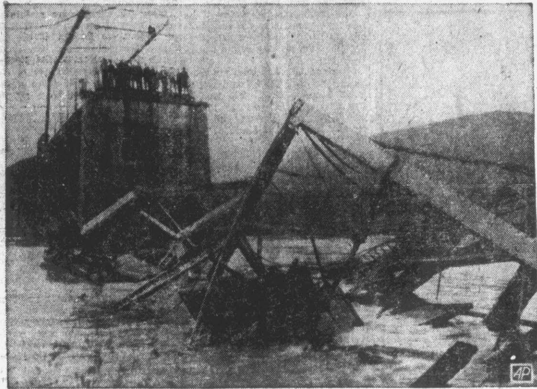
Standing on wreckage awaiting rescue by boat are three men who were crossing in an automobile when this bridge fell into the Hiwassee river near Denton, Tenn. A truck also went down with the bridge and it submerged in the flooded stream. When this picture was made, the truck driver had not been found and it was presumed he perished. (AP Wirephoto).
