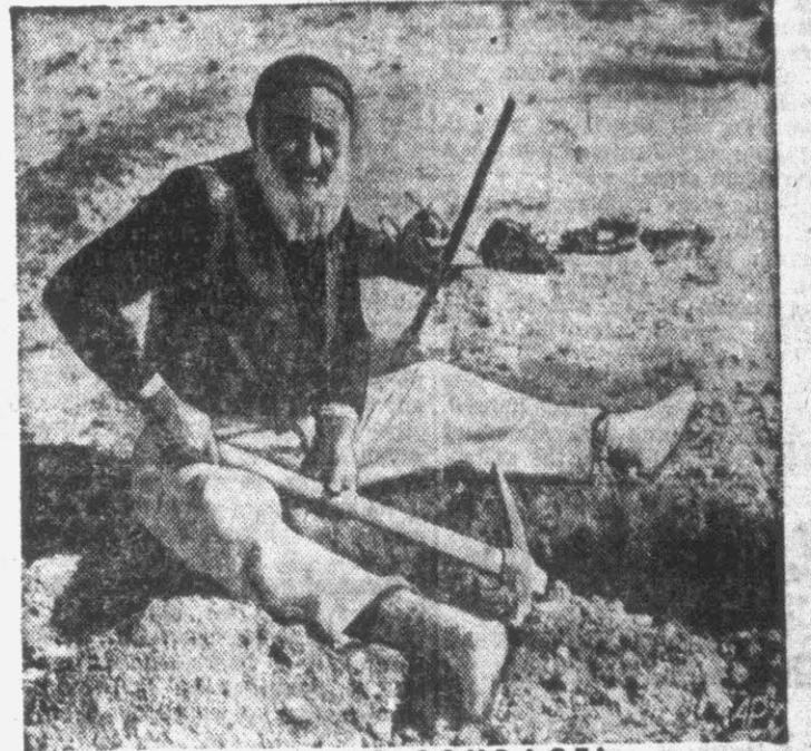
ON THE 'ROAD OF COURAGE' —An elderly Jew takes a rest from his digging while at work on the new Jerusalem-Tel Aviv highway called the "Road of Courage."
