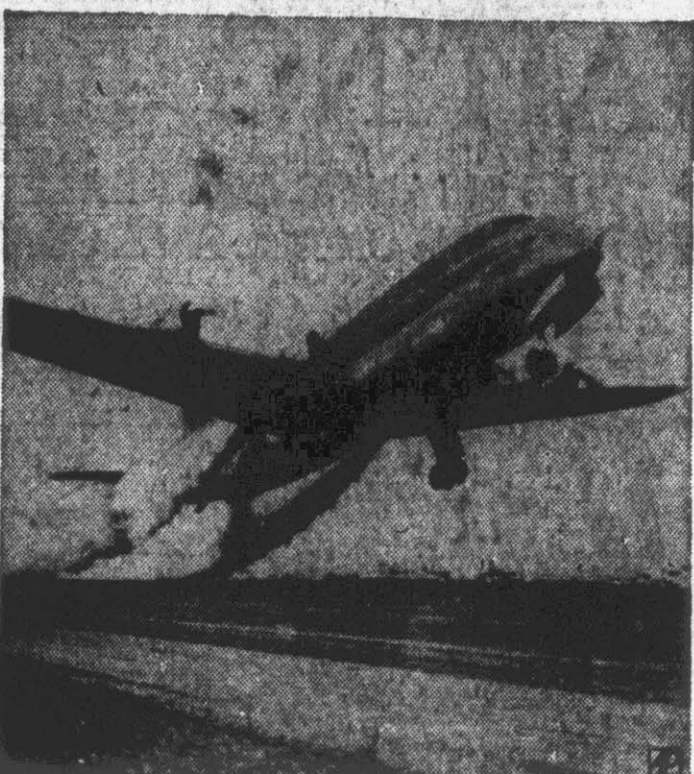
The Navy's giant 180-passenger Constitution receives terrific thrust from six rockets in takeoff at Los Angeles airfield, Burbank, Calif., in one of a series of final tests. The six JATO (jet assisted takeoff) rockets shorten the takeoff run by nearly 24 per cent. Tests were made up to 184,000 pounds gross weight on the Lockheed-built transport with the controls unaffected by the added power. Rockets give plane power roughly equivalent to one of its 3,500 horsepower engines. (AP Wirephoto).
