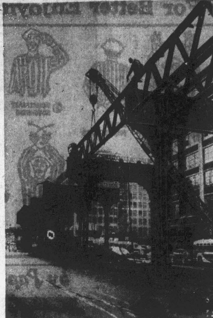
CHICAGO 'L' RAZED—Workmen apply torches to beams of 54-year-old elevated spur in Chicago as the structure is razed to make way for the Wacker Drive super-highway. The quarter-mile line ran between Lake and Madison Streets.
