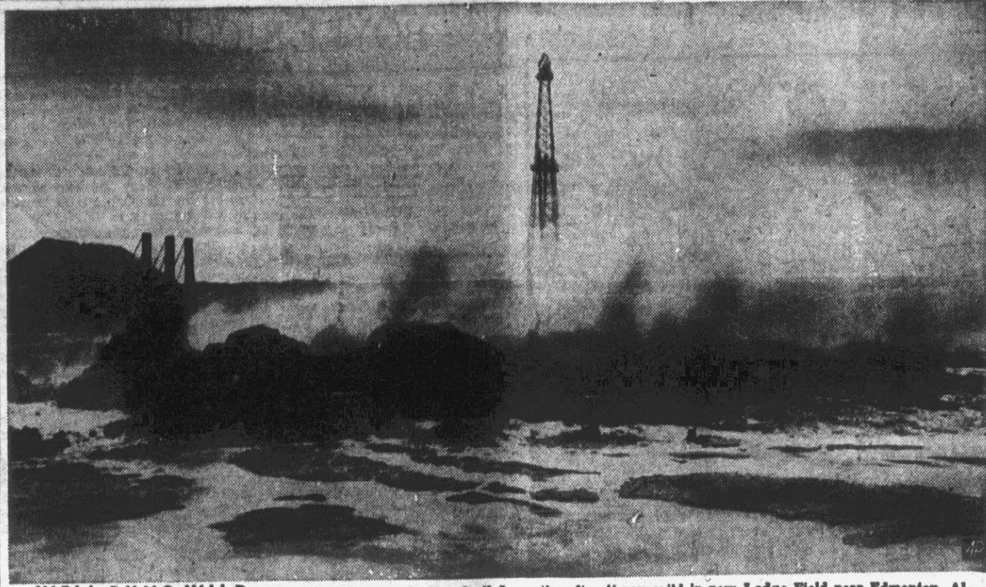
WELL RUNS WILD —Atlantic No. 3 spews gas and oil 5 months after it ran wild in new Leduc field near Edmonton, Alberta. Well has averaged 14,000 barrels daily, forming oil lake in foreground. Two-year-old field now has 100 producers.
