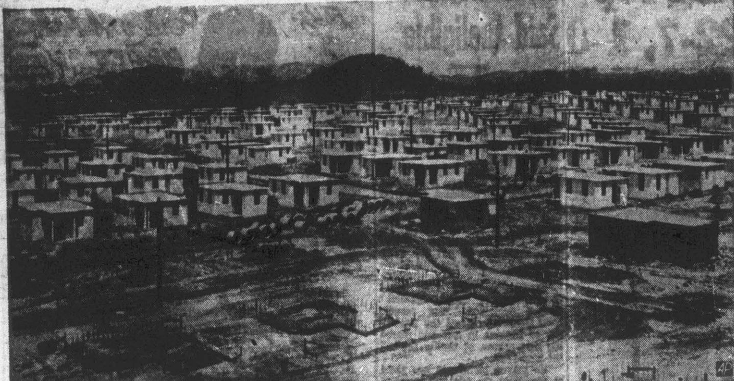
PUERTO RICO HOUSING PROJECT — These are part of 7,000 five-room concrete homes which are being built near San Juan, Puerto Rico, at the rate of 50 per day. They will sell for $4,000, with payments of $25 monthly. Non-veterans must pay $400 down; veterans nothing. The Insular Government worked out $30,000,000 project with help of Leonard D. Long, Charleston, S.C.
