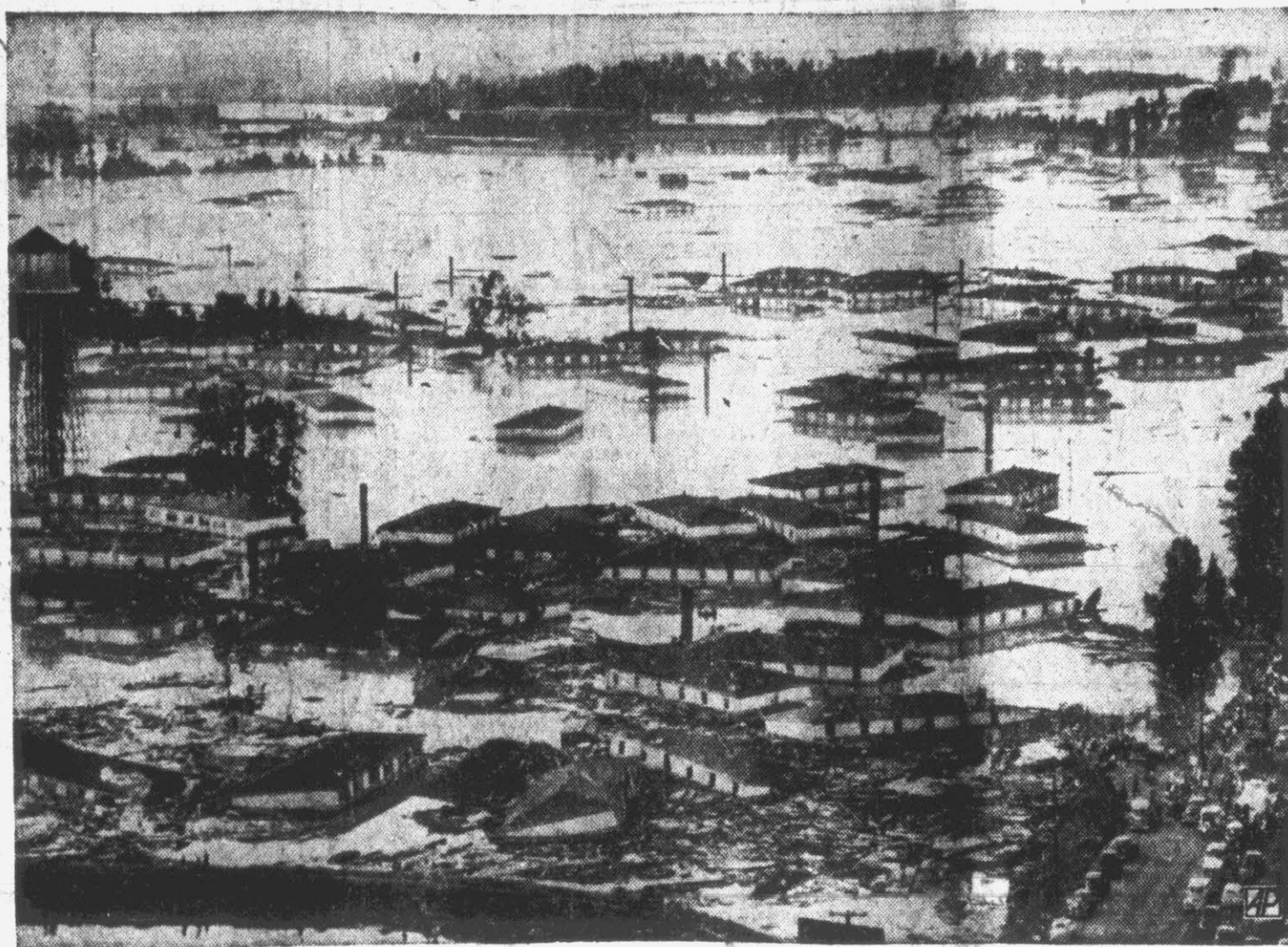
Columbia river flood water nearly covers the city of Vanport, Ore., which was destroyed within a few minutes. Only the tops of buildings remain above the surface of the water. The war-built city with a population of 18,700 is regarded as a total loss. Hundreds of rescue workers are searching for dead and injured. (AP) Wirephoto.
