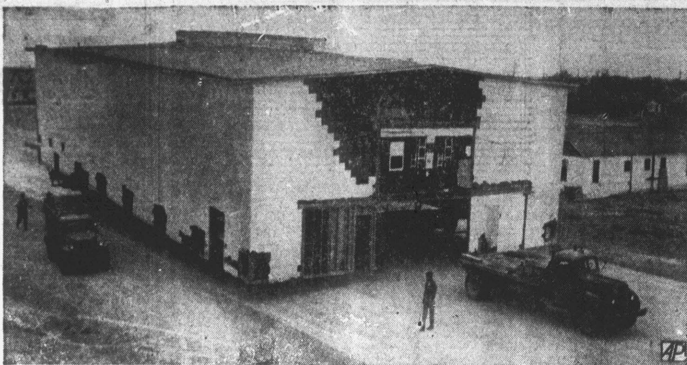
BIG MOVING JOB —The 15,000-ton building which formerly was a movie theatre at the Pecos, Tex., Airbase is moved three miles into the city of Pecos for municipal auditorium. Equipment used included 24 nose wheels from B-29 planes.
