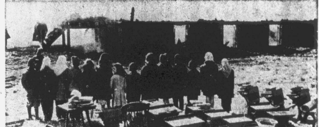
. . . . . an explosion tears the building apart
