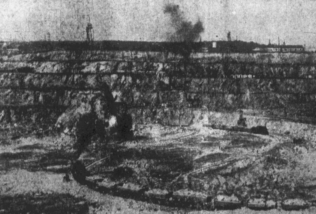
MILE-WIDE ASBESTOS MINE —Railway trains haul asbestos along 2½ miles of track in this mine—a mile wide and nearly 250 feet deep—at the settlement called Asbestos, in the Canadian province of Quebec.
